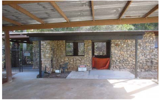
The former kiosk (work in progress) – Cammoo Caves
