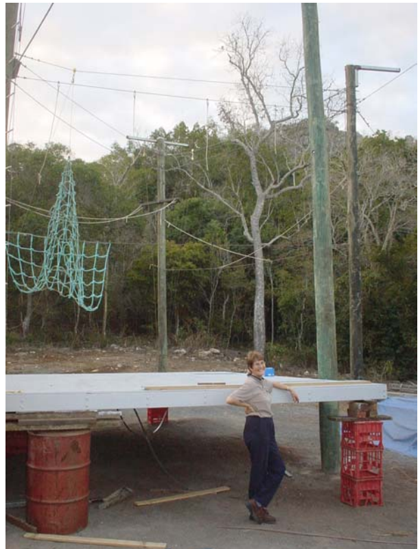
Ann Augusteyn at the new outdoor adventure area (under construction) – Capricorn Caves
